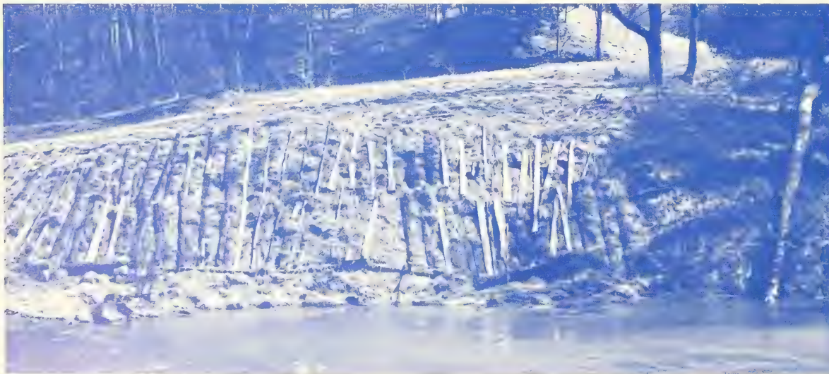
Completion of a streambank stabilization job with mulch and poles in place to stabilize the bank until vegetation covers the site.
